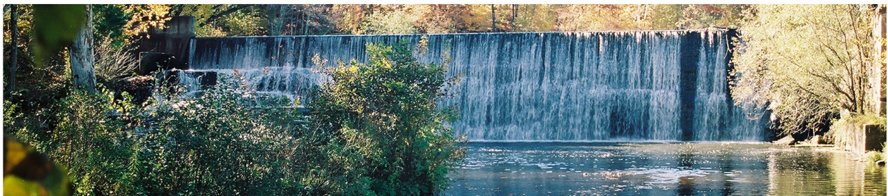
Merrillan Dam - Merrillan
